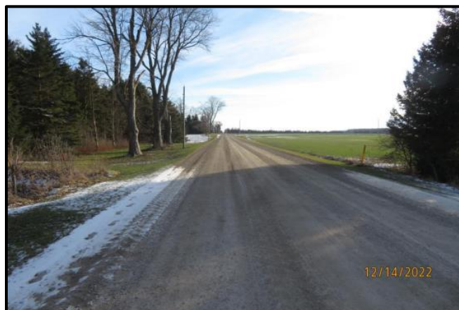
Cherry Hill Road Culvert – No. 134 (BCI = 71 Good)
