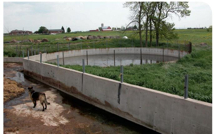
**Figure 39.** A solid, uncovered outdoor storage with uncovered liquid runoff storage (L1).
