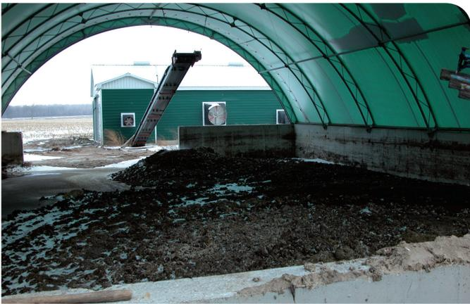
**Figure 43.** Front view of a roofed liquid storage facility (M2).
